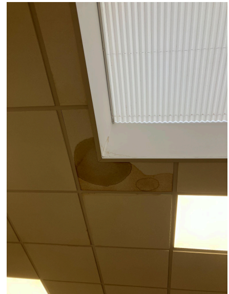
Image 7 - damaged ceiling tile in waiting room
